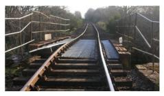
Track distortion due to a bridge strike
